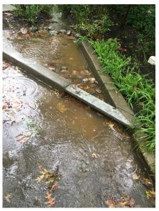
However, the *right* photo shows a rain garden that is not receiving any water from the street because the cement strip under the metal entryway arch is too high. You can see all the water, even in such heavy rain, flowing down the street toward the already overloaded Plum Run, which would benefit from receiving less runoff. The Borough has recently put a lot of effort into protecting and reinforcing its banks, and any such remediation is tenuous.
